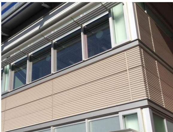
Figure 19. Corrugated metal panels
